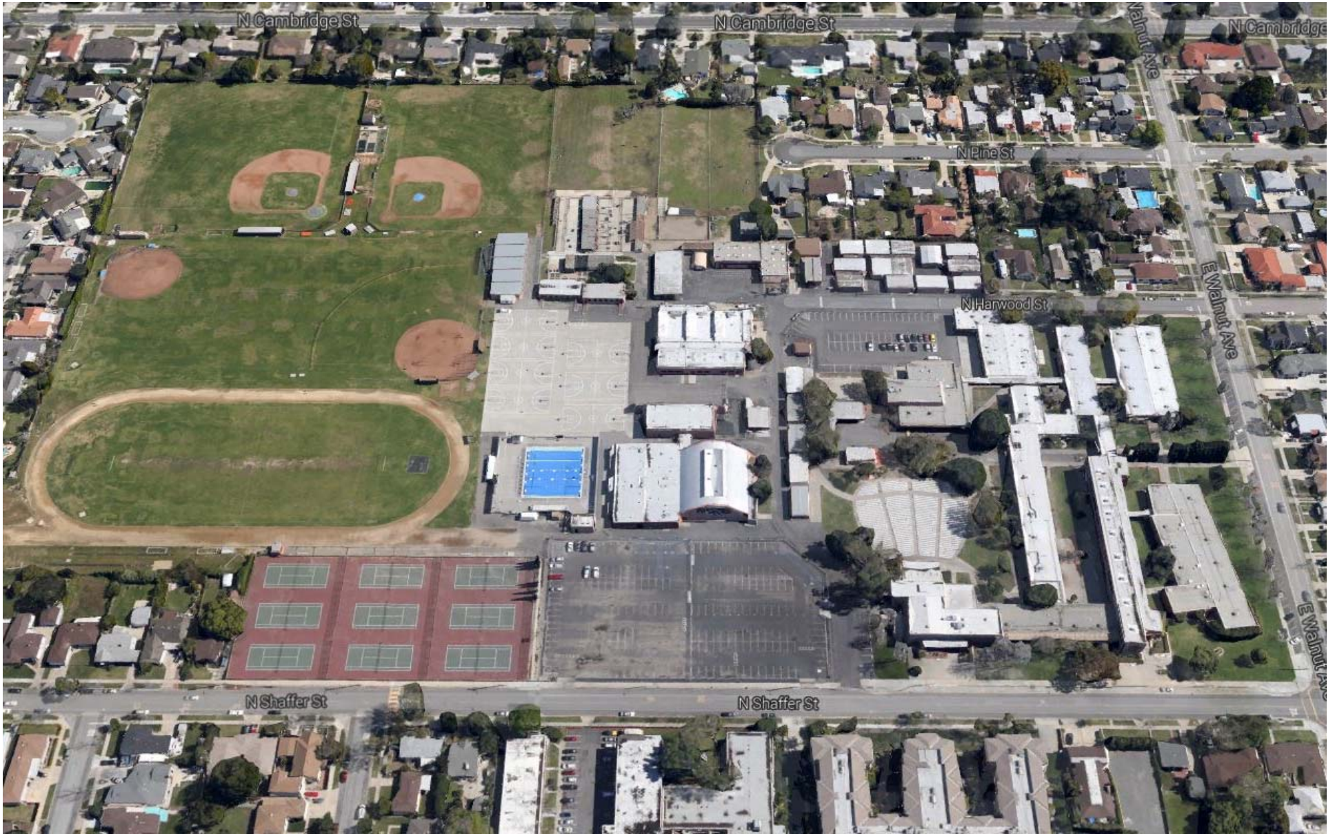
View of Existing Site
